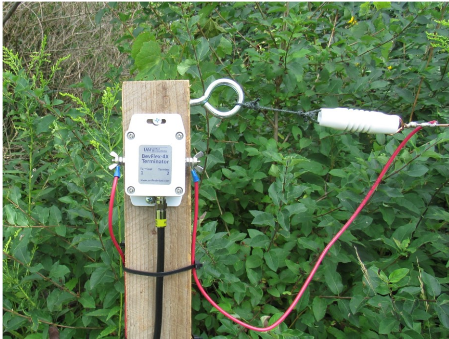
Figure 2. Proper Terminal Unit mounting. Wires and coax must come from below the Terminal so water runs away from the connections. Wires must have stress reliefs if they will put tension on the connectors. Wires coming from the side or from above must have a drip loop. Weather proof the connections. Coax connections to the Feed Unit must also drop down. Use drip loops where necessary on the RG-6 coax
